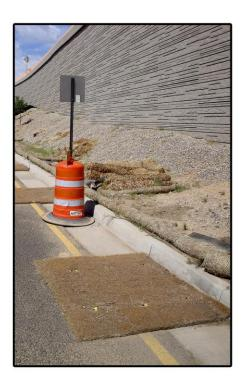
Inlet Filter serves as an excellent storm water silt filter at sewer inlets during the construction phase.
