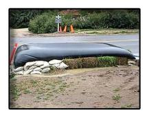
The Dandy Dewatering Bag is designed to control sediment discharge in dewatering applications where water is being pumped. When pumped water reaches the Dandy Dewatering Bag, the suspended solids are allowed to settle out of the slowed flow and are captured by the bag. Hassle free and very convenient.
